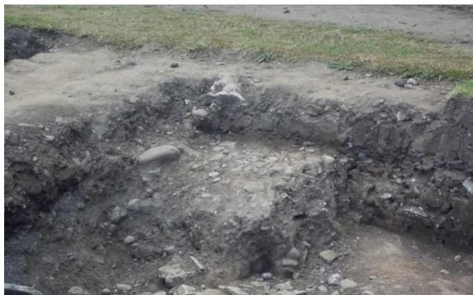
Earth Steps can also be cut into the edge of the trench which can help certain physical conditions, to access the trench.
